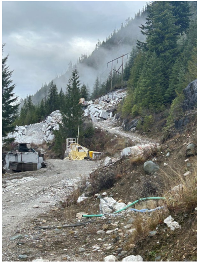
View of quarry, looking north
