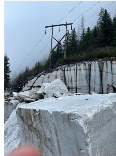
Transmission lines above quarry
